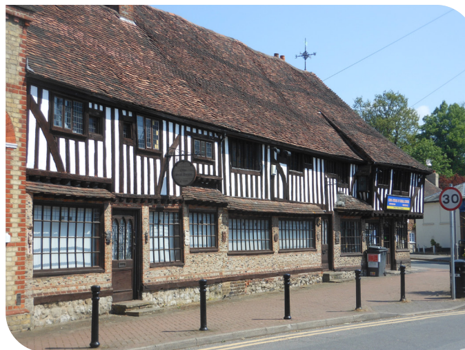
The District has a tradition of buildings made of oak frames, with painted plaster panels
