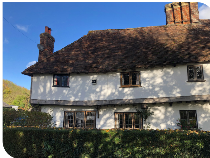
Lime render has been applied to buildings for centuries, in this case to a timber-framed house
