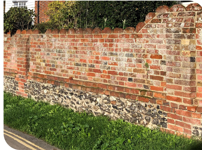
Boundary wall of handmade brick, with knapped flint base and decorative copers
