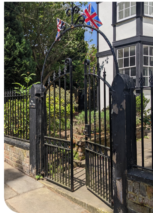
Nineteenth century cast-iron railings and gates
