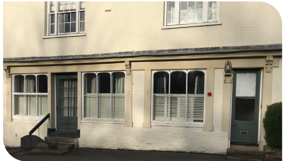
Historic shopfront, carefully retained
