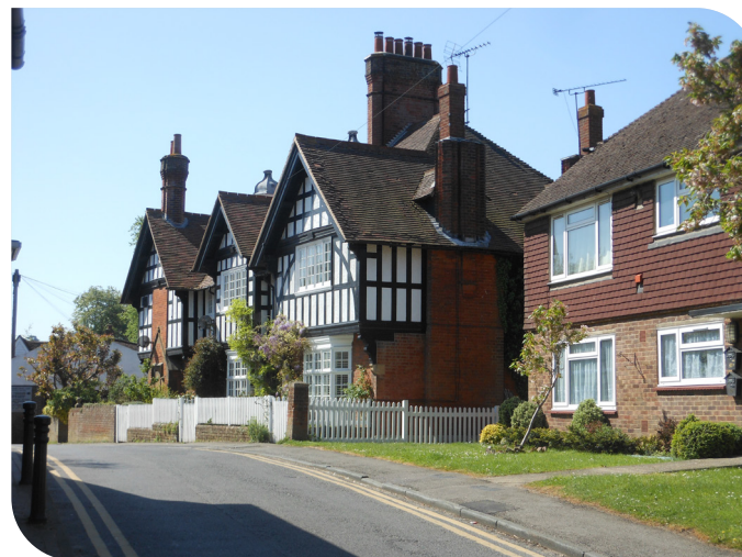
'Vernacular Revival'. Note the materials, white painted timber windows and the lively roofline
