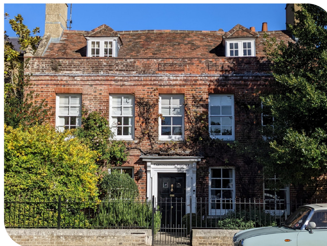
Handmade brick, with flush lime pointing
